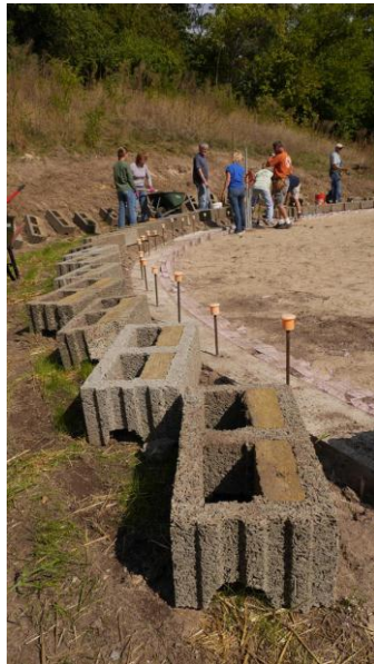
Faswall blocks made from recycled wood pallets.
